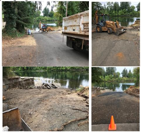
ANWS MVC procured materials, scheduled volunteer work parties to install forms and reinforcing steel to ensure the longevity of this new ramp. This physical work took two days (August 14 & 15) and allowed the City to inspect the reinforcing bars prior to being covered with cement.
