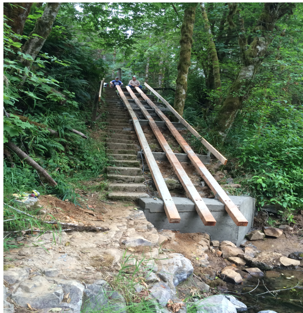
Slide lengthened, side guide board raised and secured, and large concrete base installed & pinned to the bedrock to prevent erosion, new cable and block pulley installed.
