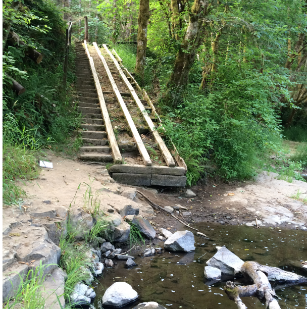
Bottom support was being eroded and boards were falling apart.
